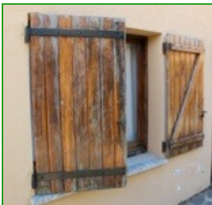
Porticons a rehabilitar
